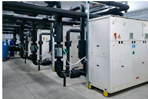
Water-to-water heat pumps at the MAHLE plant in Aleksandrovac
